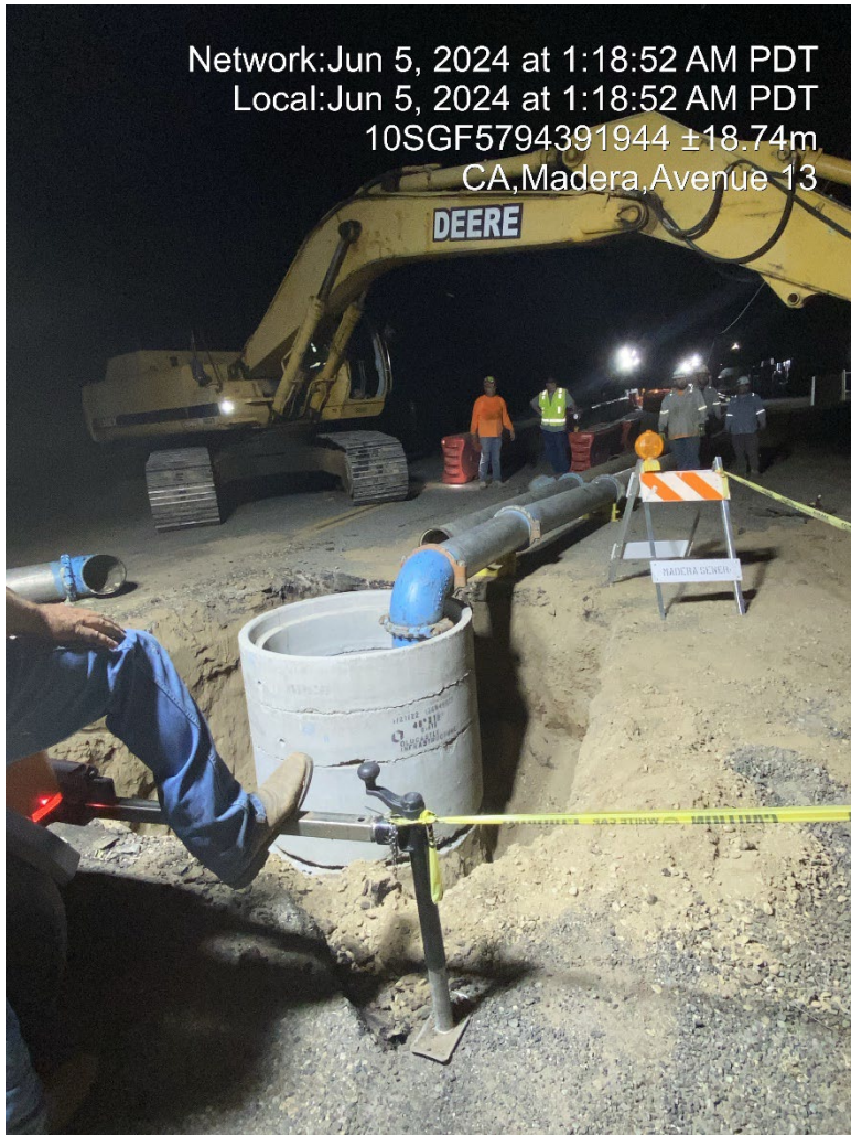
Bypass Pumping Set Up
