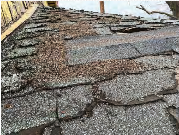
Composition Shingle Roofing
