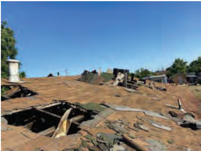
Rolled Composition Roofing – House Two
