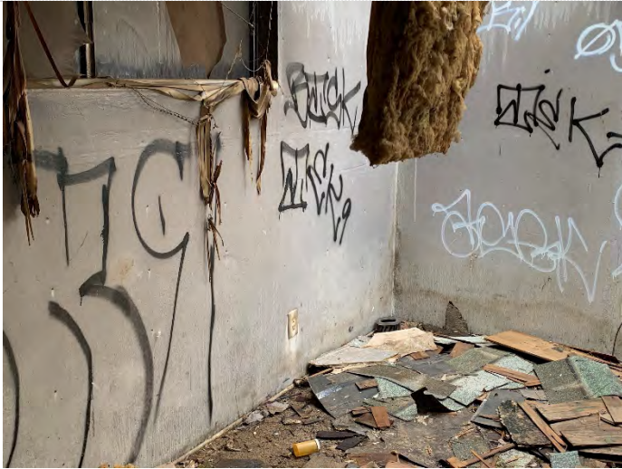
Drywall Main House
