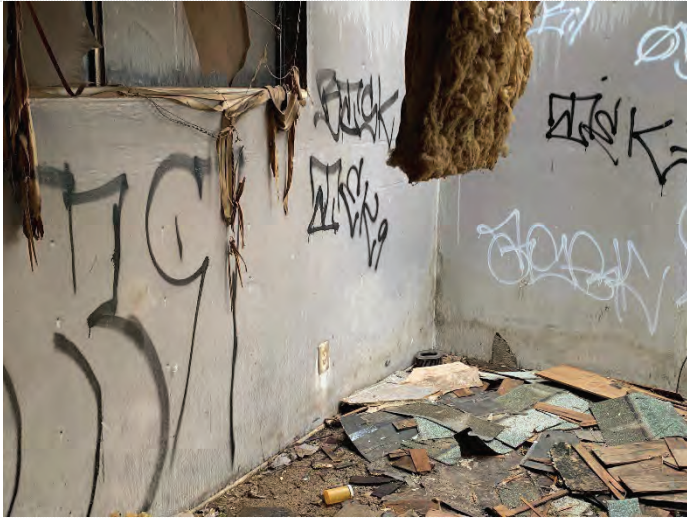
Drywall Main House
