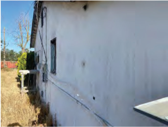
Stucco – House Two
