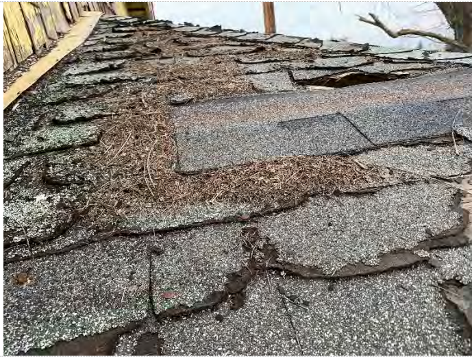
Composition Shingle Roofing
