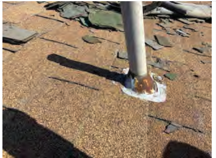
Penetration Mastic – Grey – House Two
