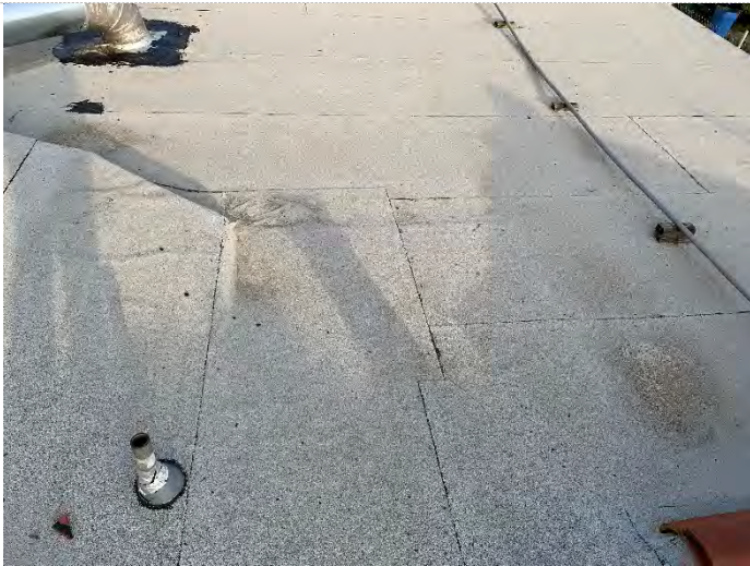
Rolled Composition Roofing
