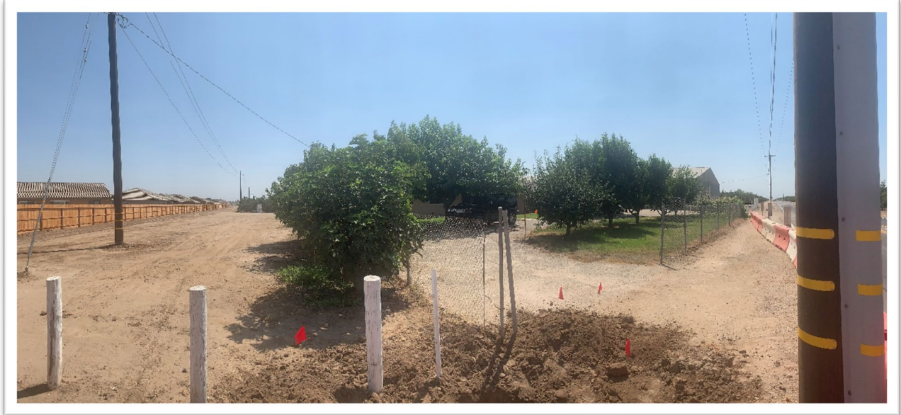
Source: Precision Civil Engineering, image captured August 2021
