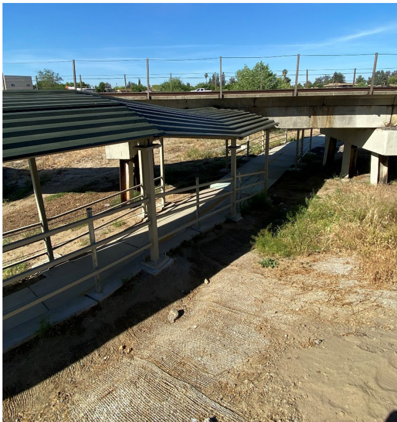
Figure 3: AFTER - east side of UPRR bridge looking west
