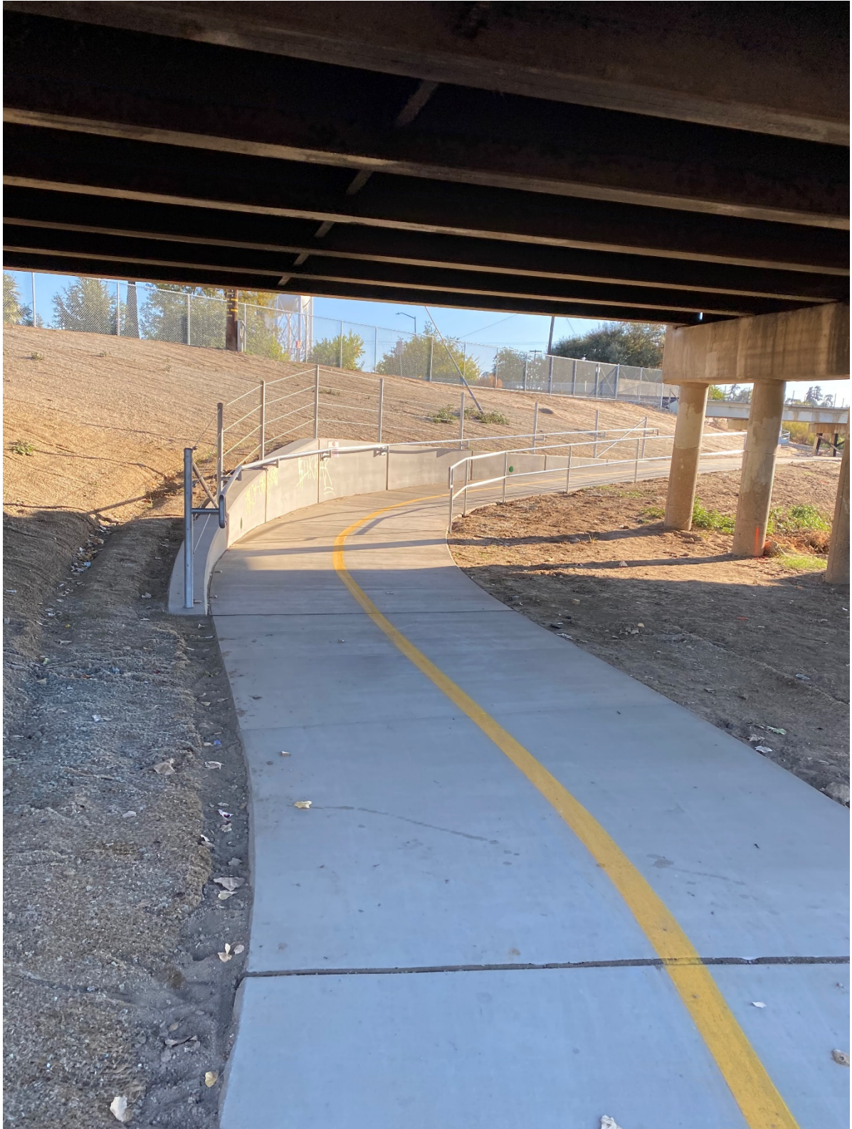
Figure 4: Looking east under Gateway Bridge
