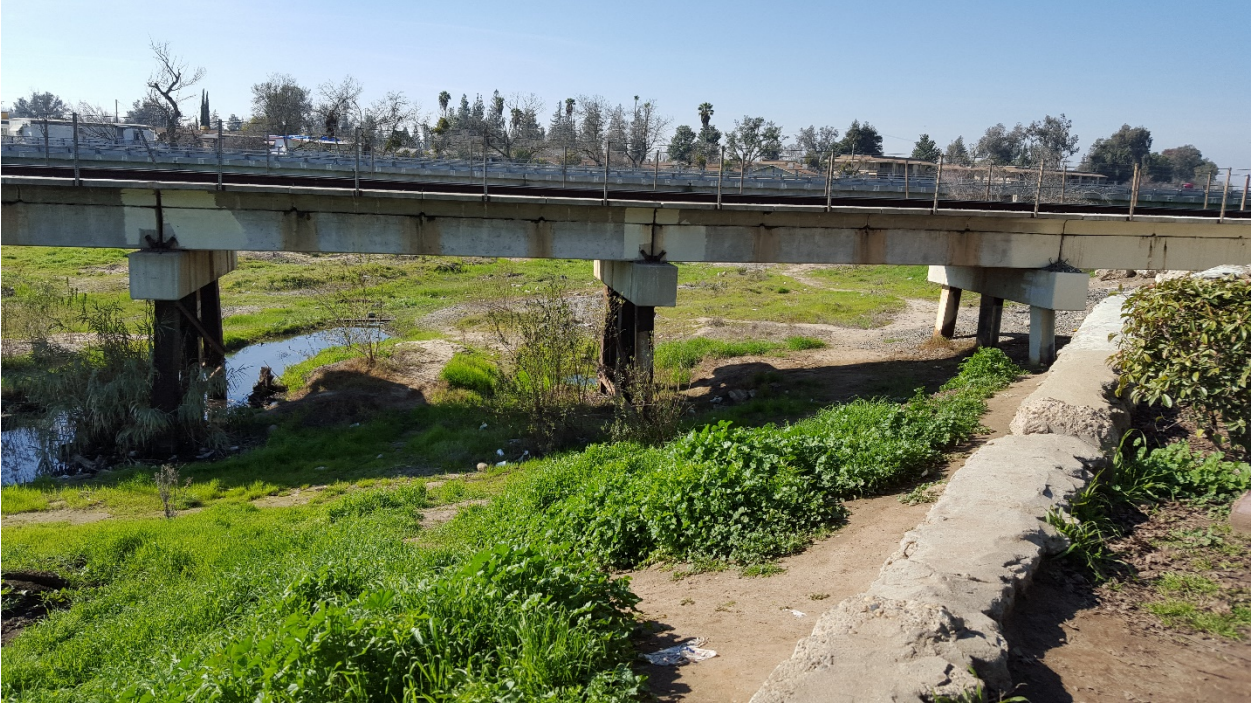
Figure 2: BEFORE - east side of UPRR bridge looking west
