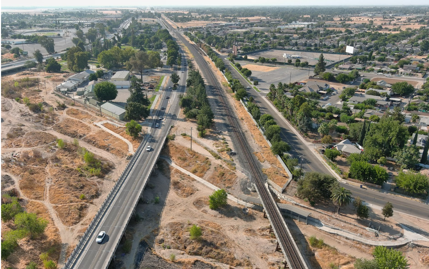
Figure 1: Aerial View of Completed Project.
