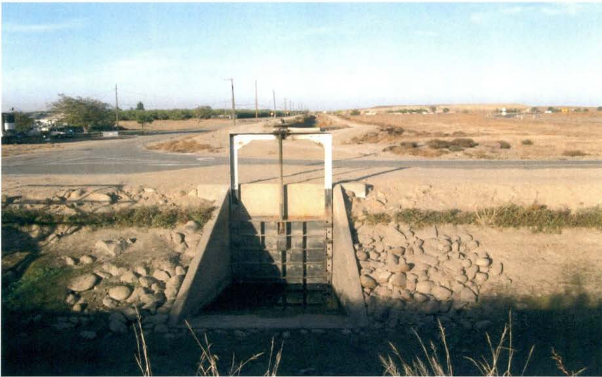
Figure 1 11/2/13 8:36 #13 Lateral 32.2-9.9 Head Overview 14 IMG-0027 west
