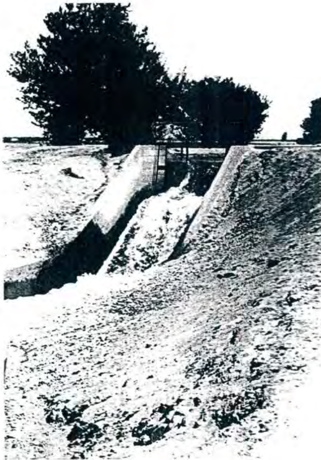
Feature 9: Lateral 32.2-9.9 Drop Structure (view looking north)
