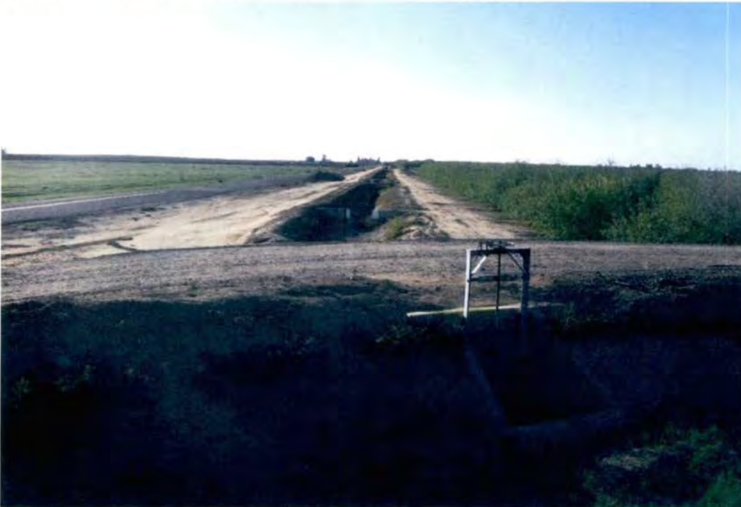
Figure 10 Lateral 32.2-9.9-6.5 overview west IMG-0578
