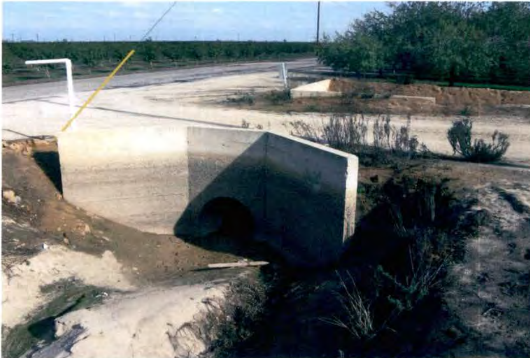
Figure 7 Lateral 24.17.0 canal siphon ne corner GPS point 2 east IMG-0600
