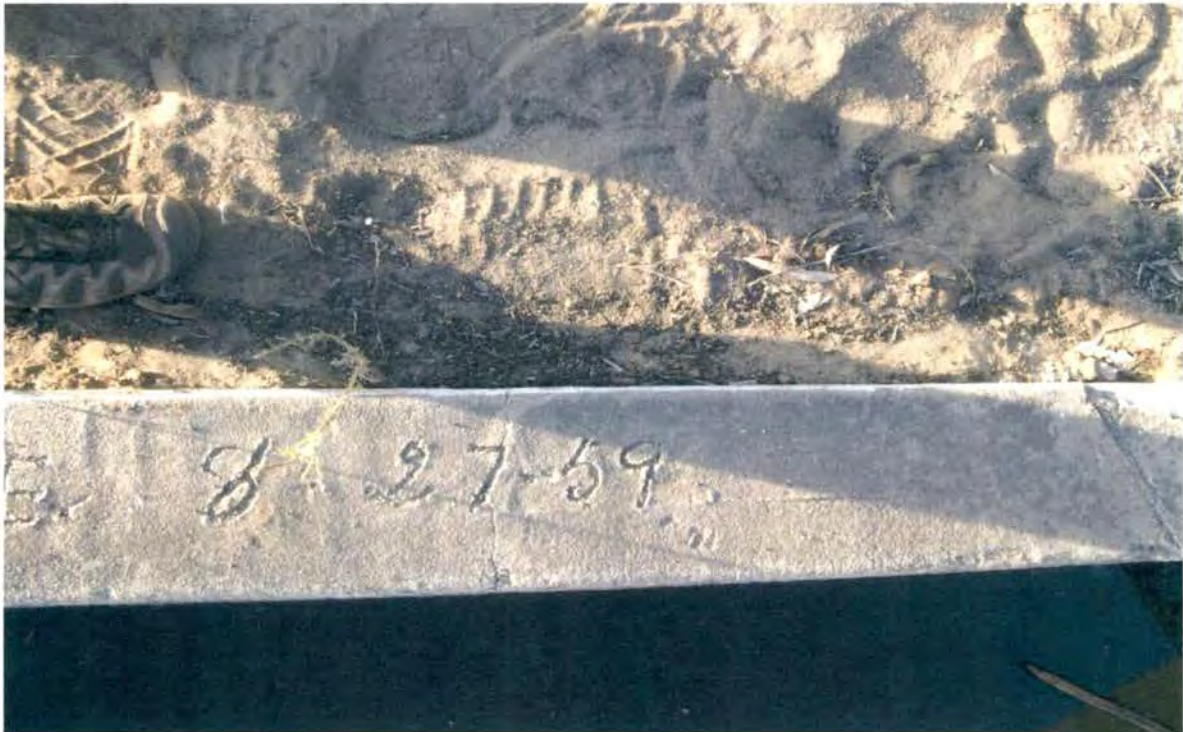
Figure 12 10/4/13 5:35 #3 Main I Head dates in wing wall "1959" 12 IMG-0012 detail
