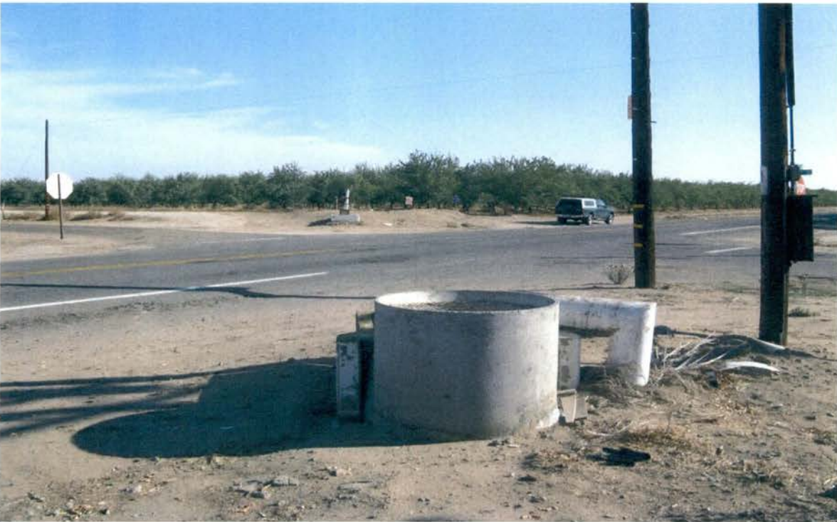
Figure 14 11/2/13 10:50 #20 Downstream Lateral 32.2 Basin Overview 27 IMG-0040 50°
