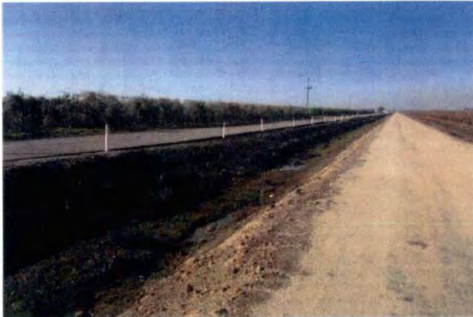
Figure 2 Segment of MID Lateral 6.2-9.2, south of Avenue 8 in Madera County
