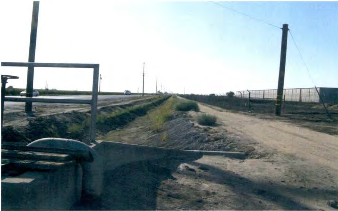
Figure 3 10/4/13 3:45 #6 Butin Head Canal Overview 3 IMG-0003 West
