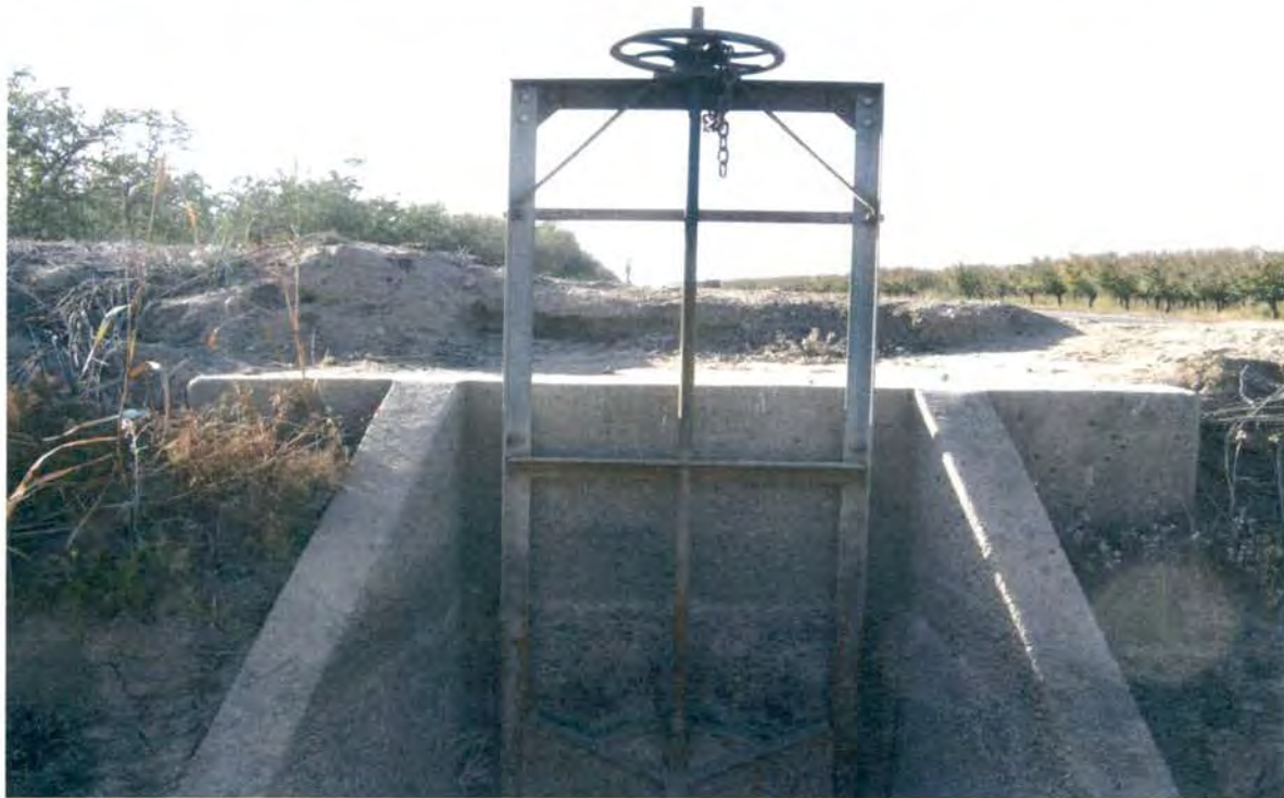
Figure 8 11/2/13 #17 Lateral 32.2-9.9 W-1.5 Head Detail 21 IMG-0034
