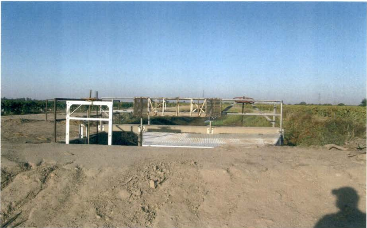
Figure 6 10/4/13 4:25 #19 Main Head II Overview 6 IMG-0006 East
