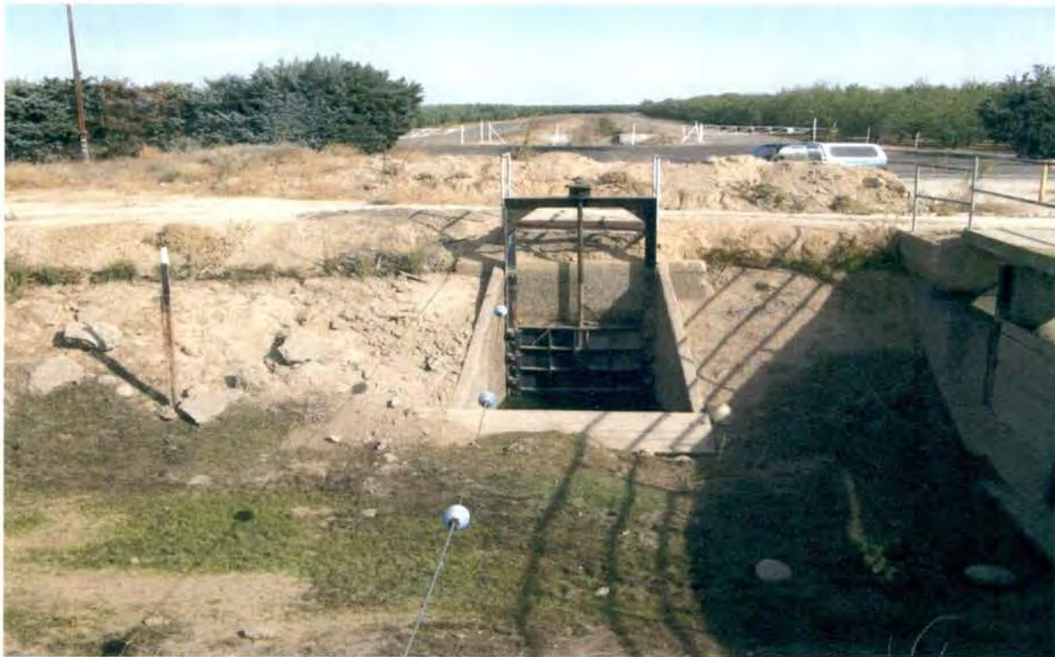
Figure 31 11/2/13 2:30 #26 Lateral 6.2-9.2 Head Overview 44 IMG-0057 east
