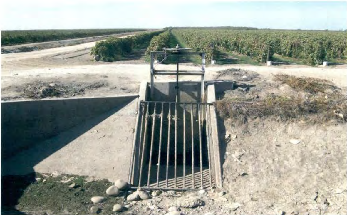
Figure 21 11/2/13 12:06 #12 Lateral 24.2-19.5 Head Overview 34 IMG-0047 west
