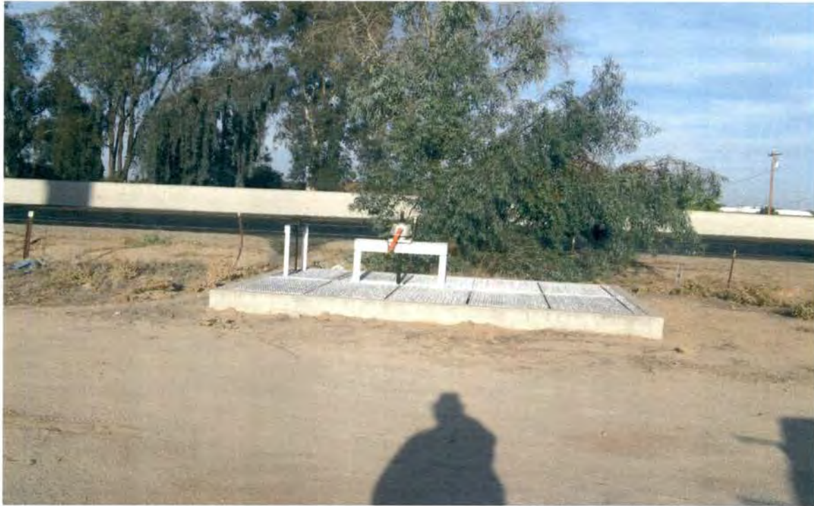
Figure 33 11/2/13 3:45 #9 Lateral 24.2-13.2 Head Overview 49 IMG-0062 east
