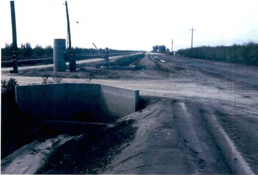
Figure 3 Lateral 24.2- 17.0 canal siphon at access road west IMG-0596
