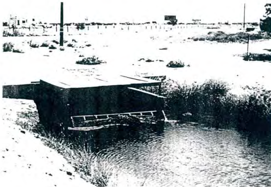
Feature 8b: Lateral 32.2 at Avenue 21 and Golden State (view looking east)
