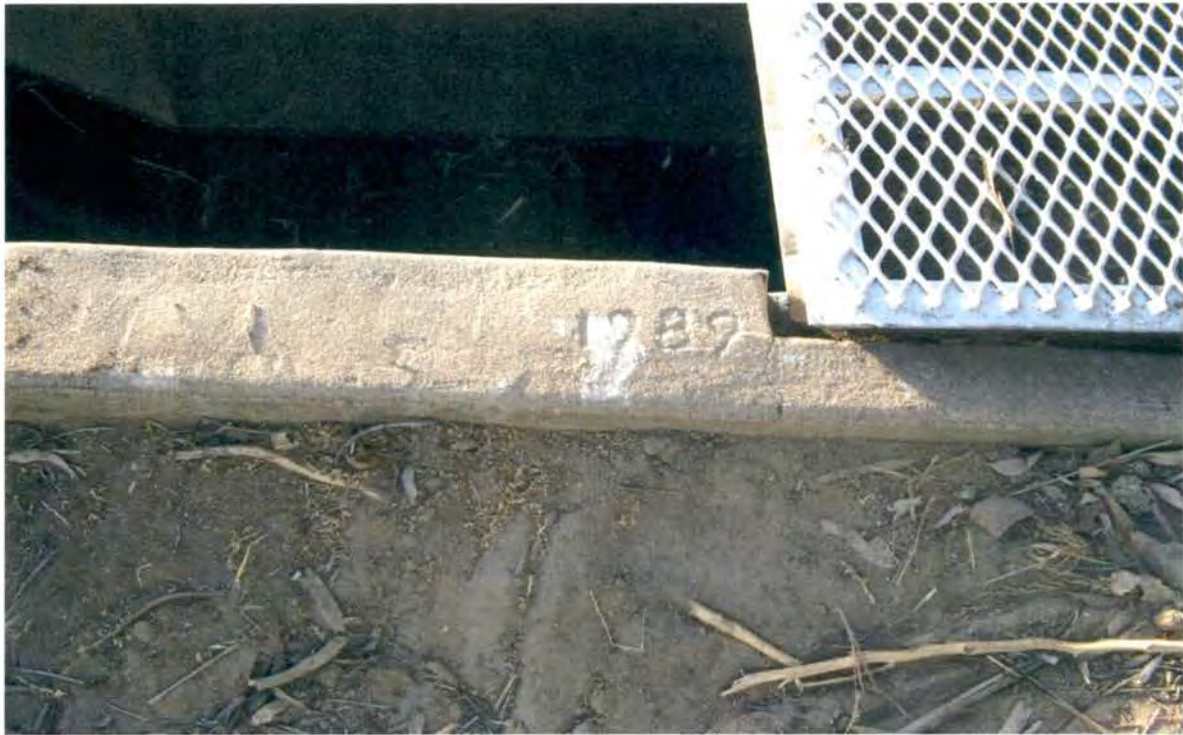
Figure 11 10/4/13 5:30 #3 Main I Head dates in wing wall "1989" 11 IMG-0011 detail
