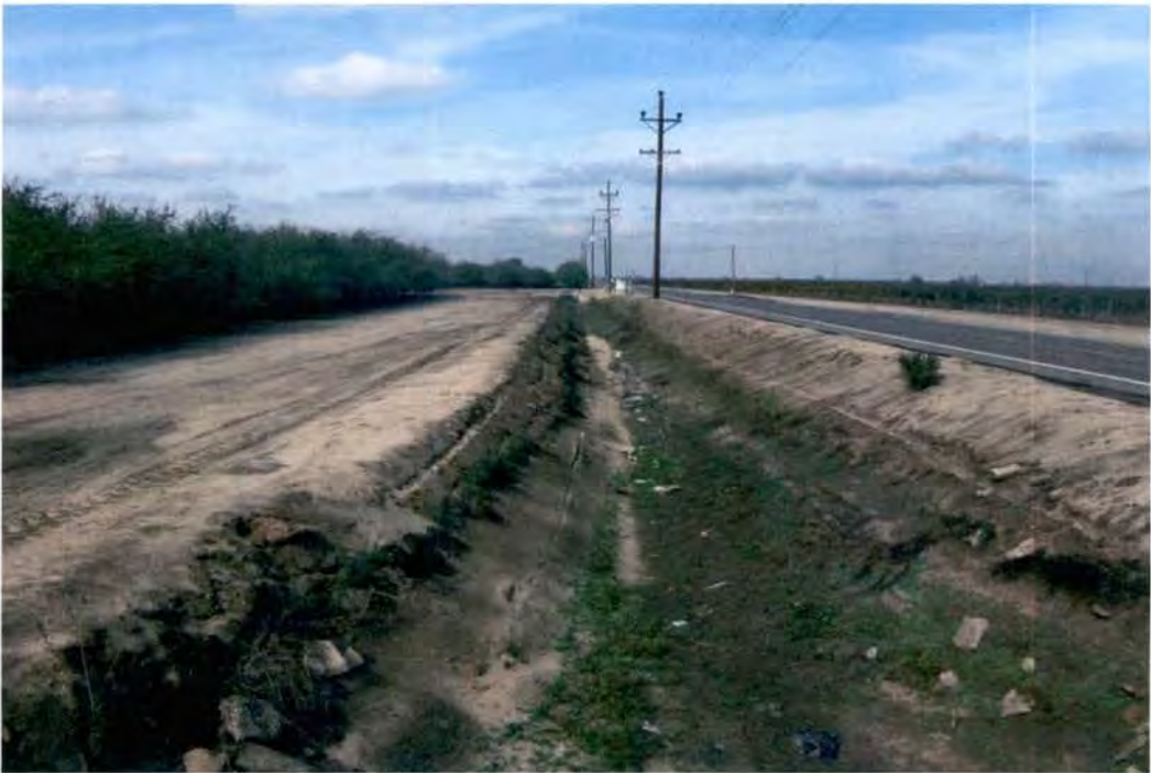
Figure 12 Lateral 24.2-17.0 canal at southeast end along Road 19 north IMG-0611
