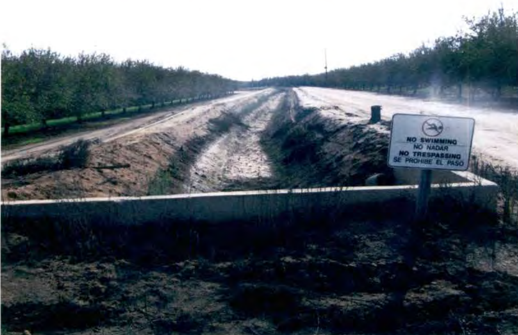
Figure 8 Lateral 24.2-17.0 canal second leg GPS point 2 south IMG-0602
