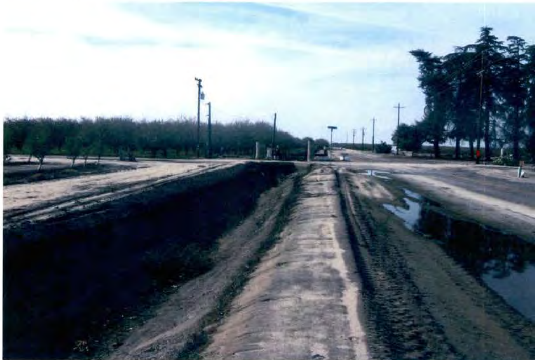
Figure 4 Lateral 24.2-17.0 canal west end at Road 18 west IMG-0597
