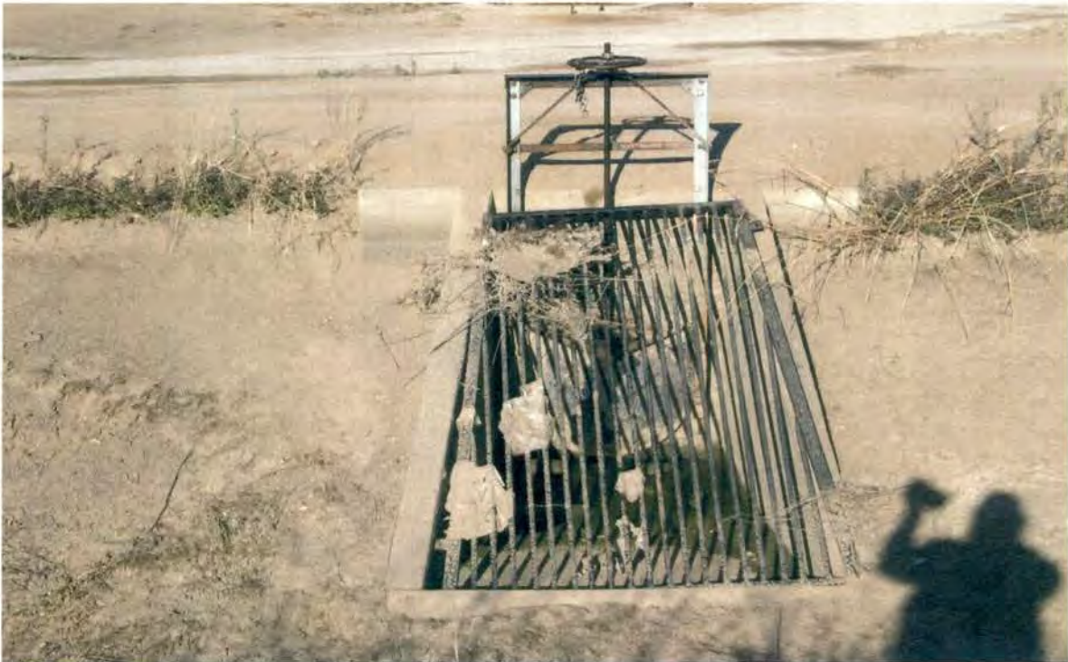
Figure 11 11/2/13 #18 Lateral 32.9-9.9 W-2.0 Head Detail 24 IMG-0037
