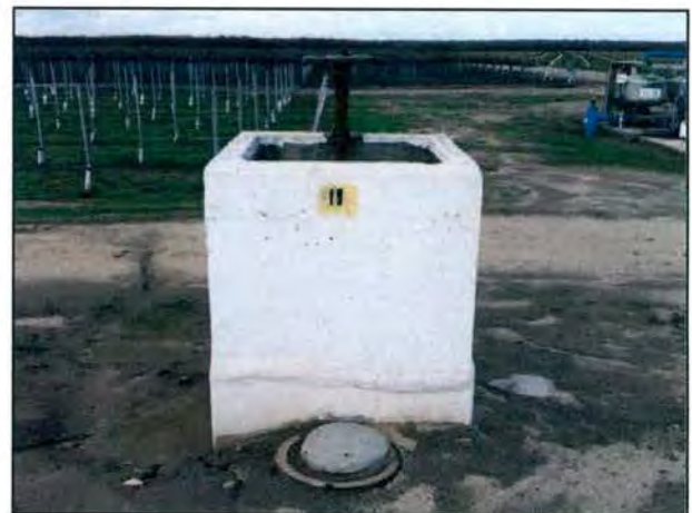
Close-up of ancillary gate and concrete housing, facing north.
