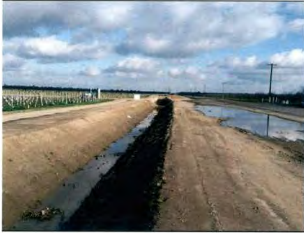
Overview of canal segment and structural components, facing east.
