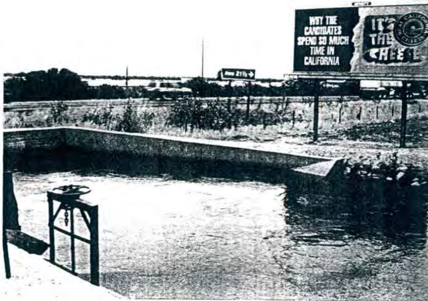
Feature 8: Lateral 32.2, West Side of SR 99 (view looking east)
