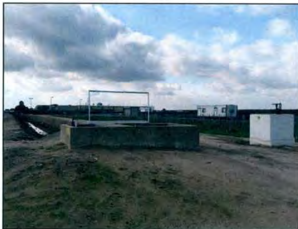
Close-up of culvert and ancillary gate, facing west.
