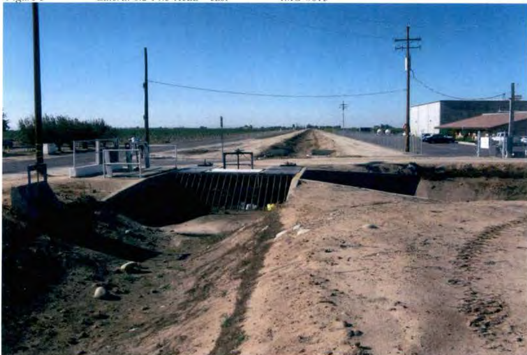
Figure 4 Lateral 6.2 15.9 overview west IMG-0549
