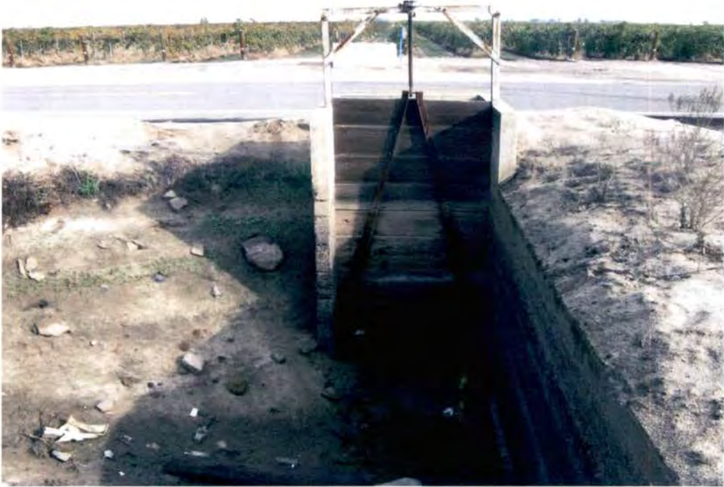
Figure 11 Lateral 24.2-17.0 canal at southeast end with slat gate east IMG-0610
