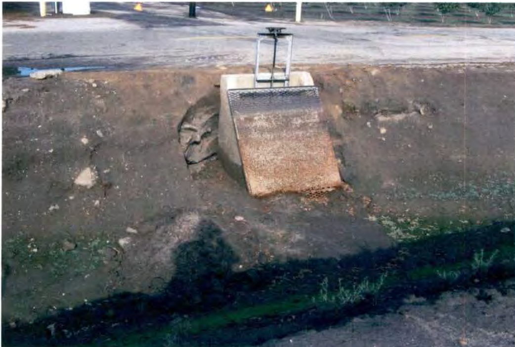
Figure 6 Lateral 24.2-17.0 canal handwork north IMG-0599
