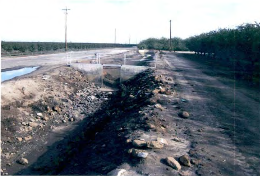
Figure 5 Lateral 24.2-17.0 canal slat dam east IMG-0598
