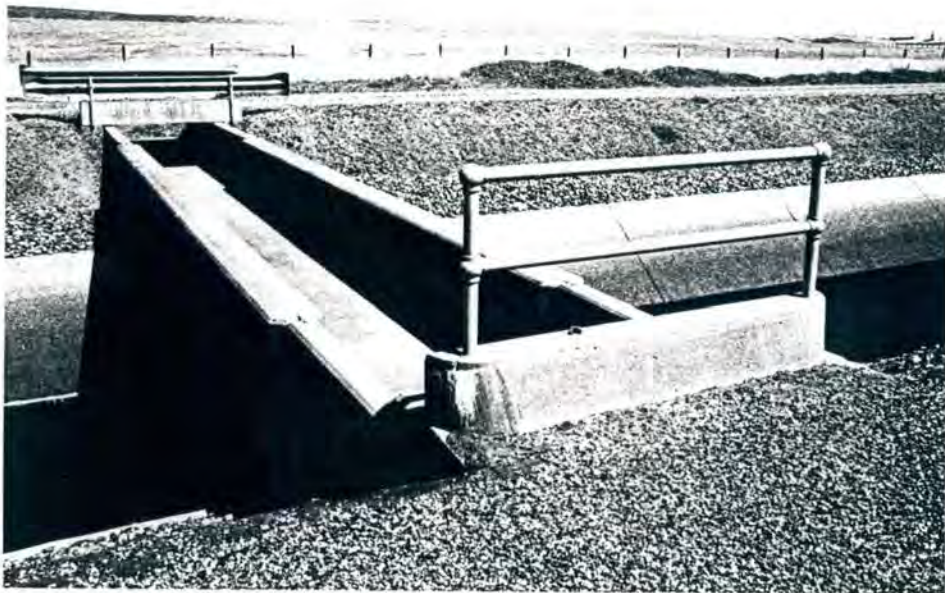
Flume across Madera Canal.
