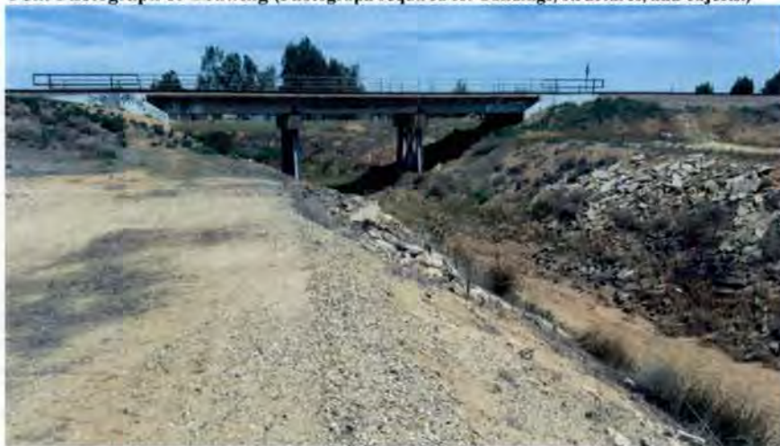
P5a. Photograph or Drawing (Photograph required for buildings, structures, and objects.)
