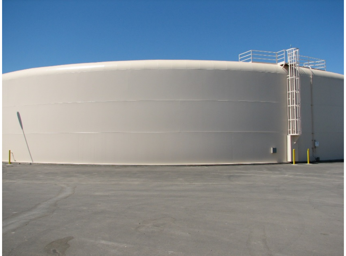
Figure 1 Welded Steel Tank
