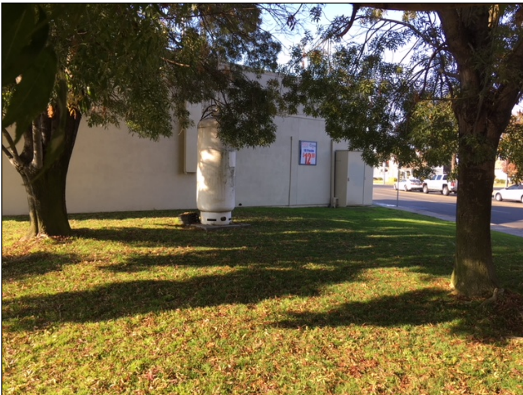
Rear of store site, with unnecessary signage.
