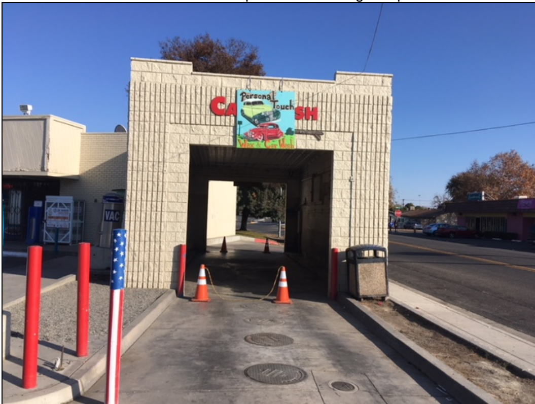
Non-operational automatic car wash with non-permitted business and signage.
