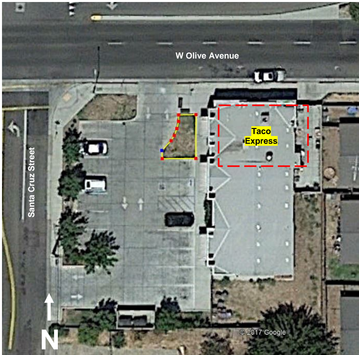
Patio area being utilized for outdoor dining
