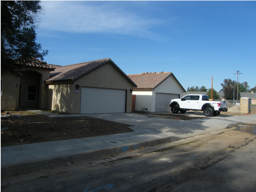
New constructed homes adjacent to project site
