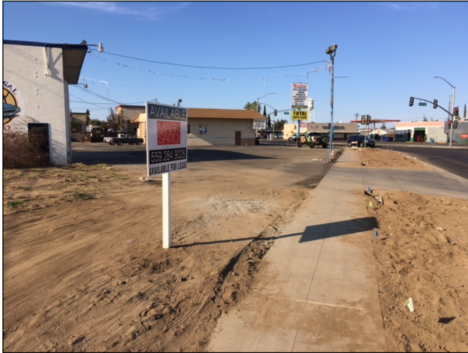
Incomplete frontage improvements along State Route 145.
