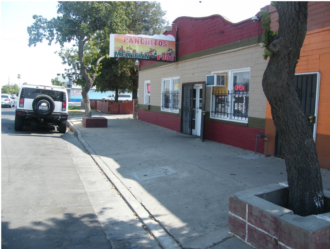
Frontage view of the site from C Street with unutilized driveway approach
