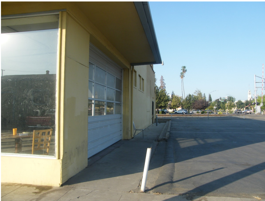
Uninstalled accessible ADA parking stalls
