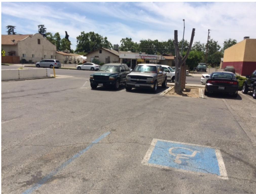
ADA parking stall is not correct. No loading zone is provided.
