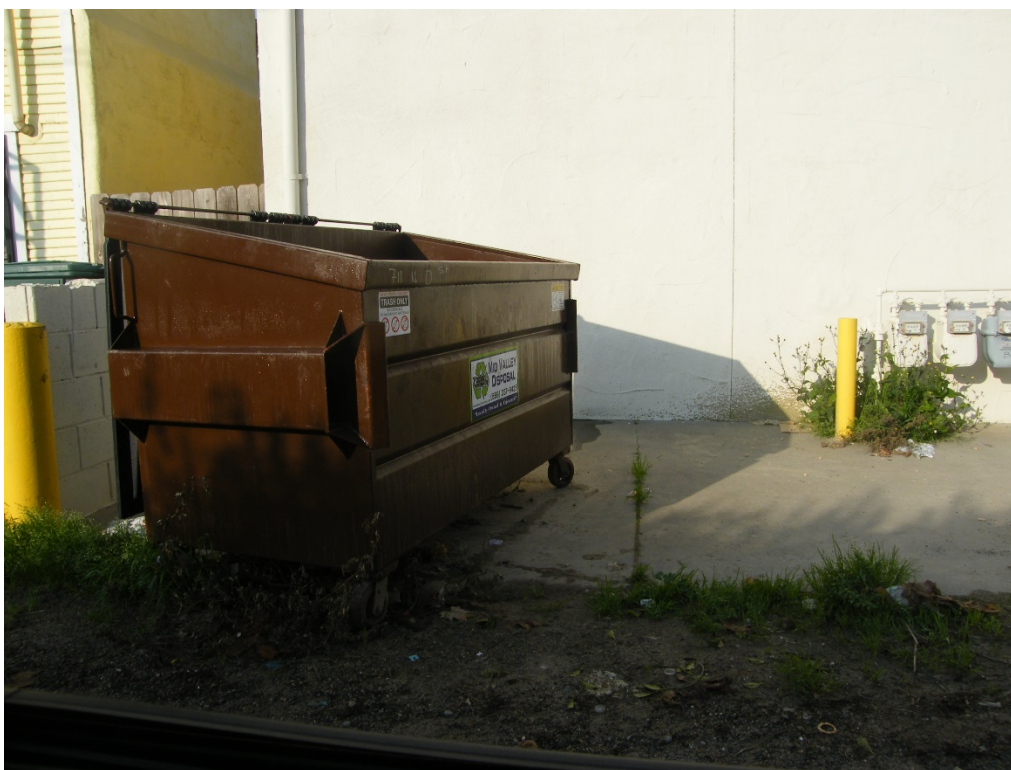
The required trash enclosure has not been constructed.
