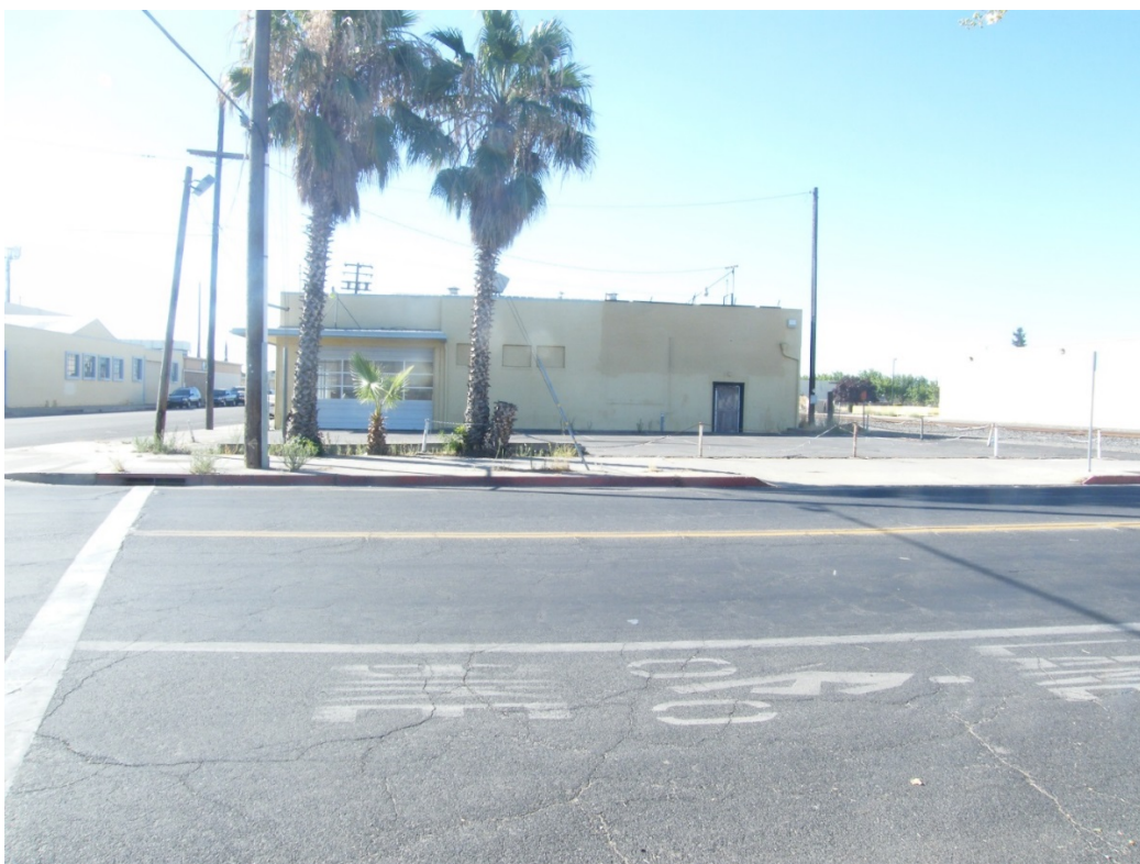
Unreconstructed driveway approaches and damaged sidewalk
