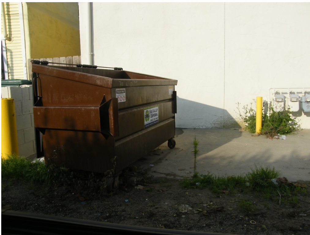
The required trash enclosure has not been constructed.
