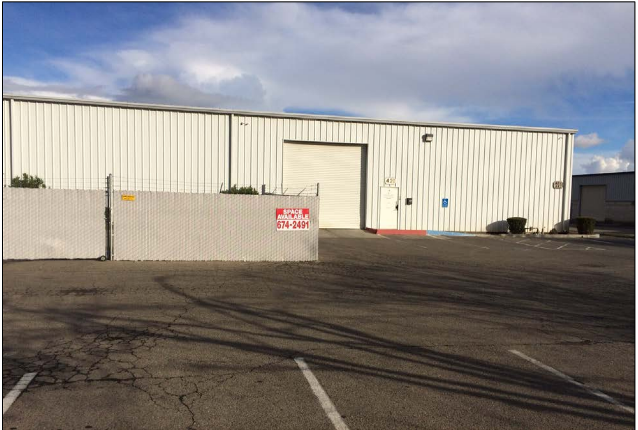
The site in January, 2017.
