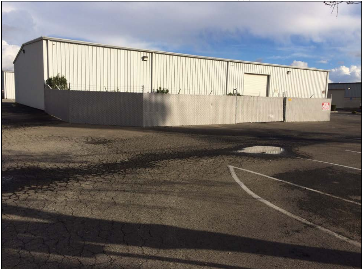
The site in January, 2017.
