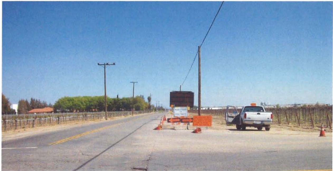
One of the pre-construction zone warnings regarding road closure: intersection of Road 23 & Pecan
