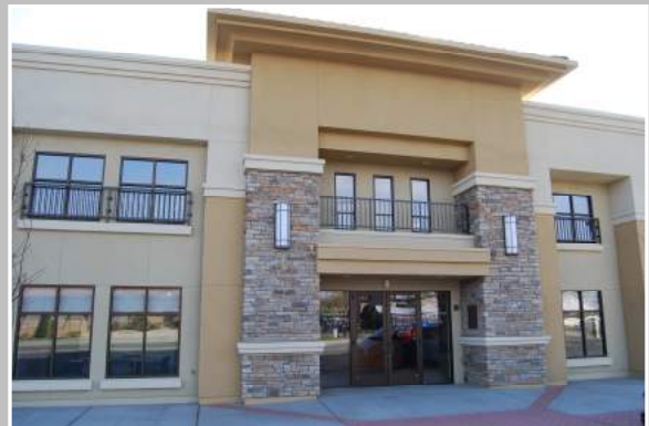
Completed Remodel Project
