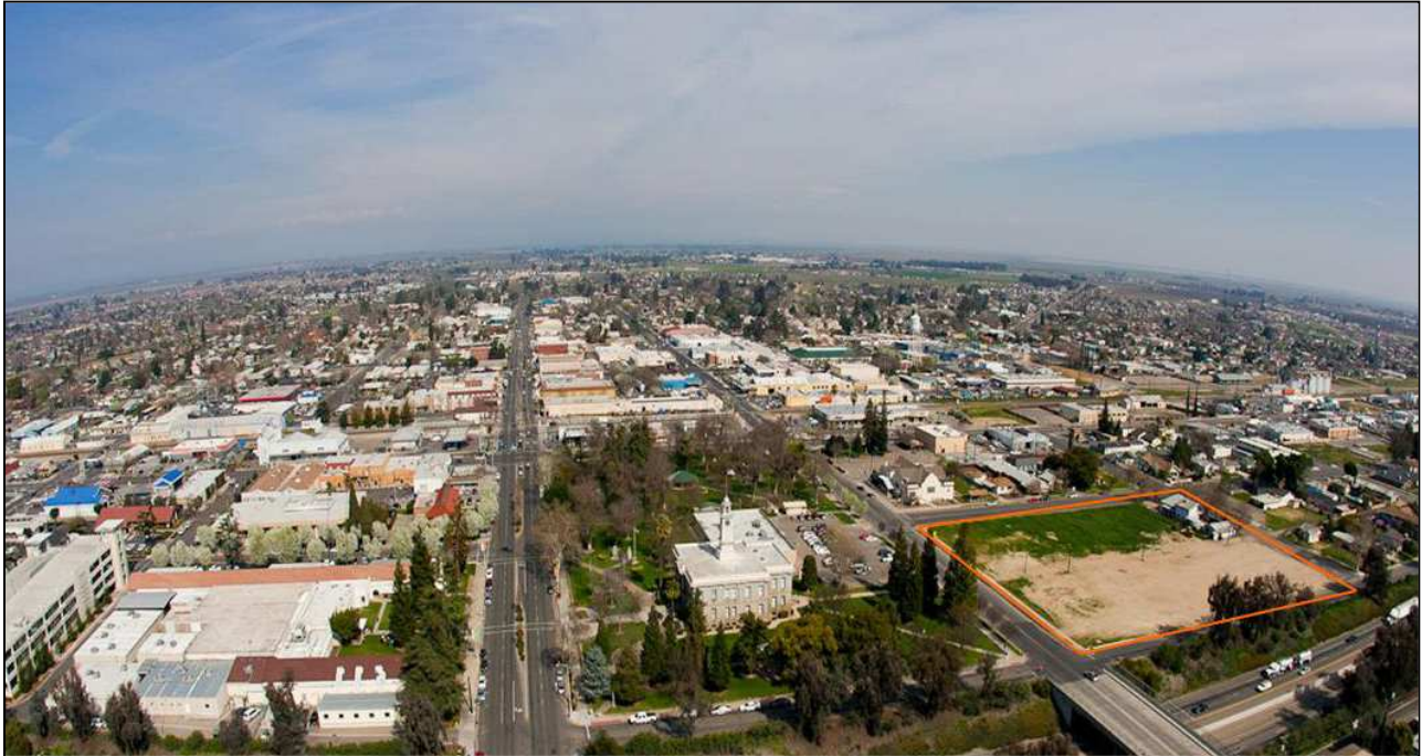
Future site of New Courthouse Facility in the lower right corner of photo
